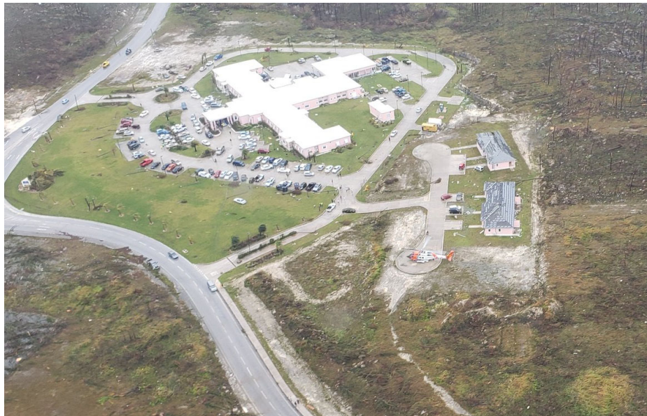
Figure 4.9. Aerial view of Marsh Harbour Healthcare Center [Located at 26.534, -77.070] and accessory buildings (a) before Hurricane Dorian and (b) afterward, exhibiting no significant structural damage. Nearby trees are debarked. (Source of pre-event image: Google Maps; Source of post-event image: U.S. Coast Guard )
