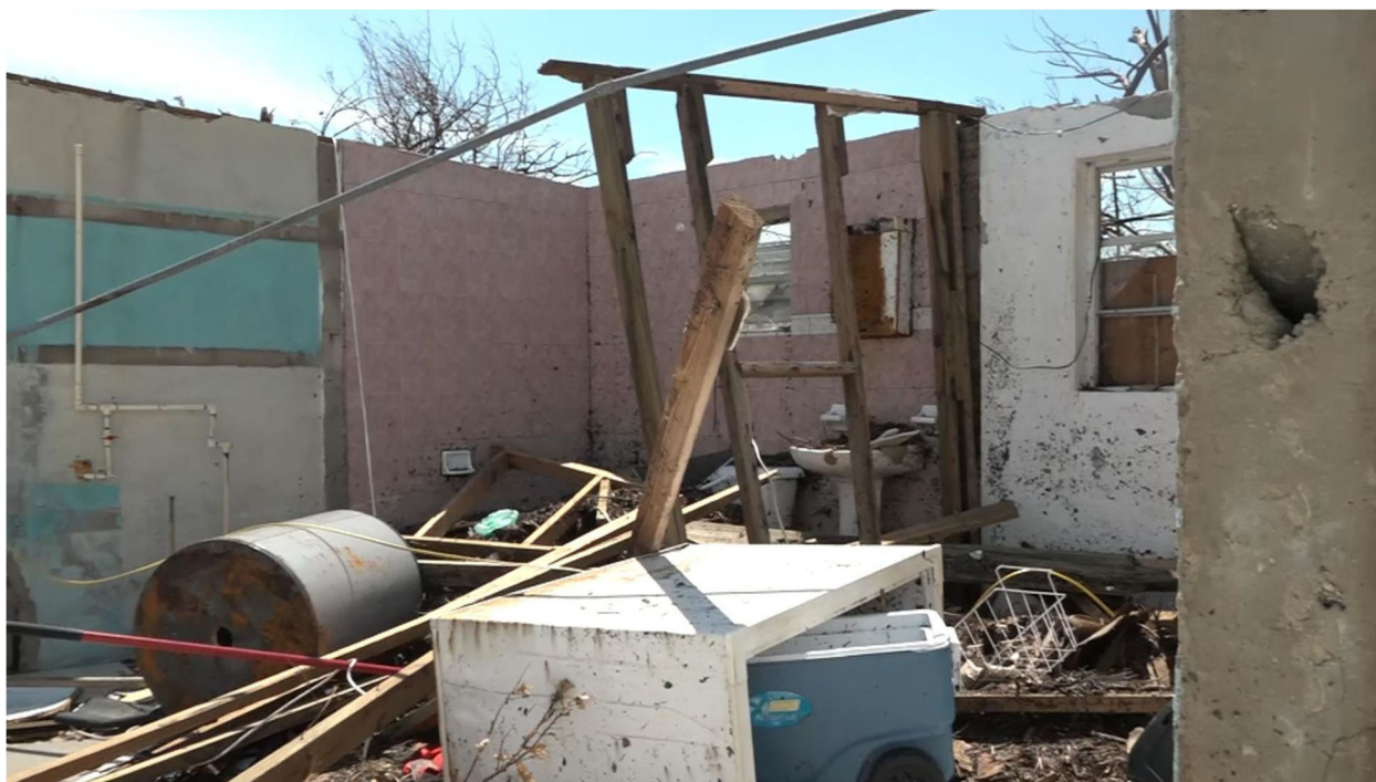
Figure 4.31. Damage to concrete/masonry residential construction in High Rock, Bahamas. (Source: SkyNews )
