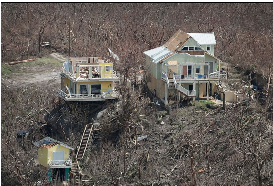
Figure 4.5. Damage to roof and walls of a pair of homes at an upper elevation on Great Abaco Island (Source: Orlando Sentinel )
