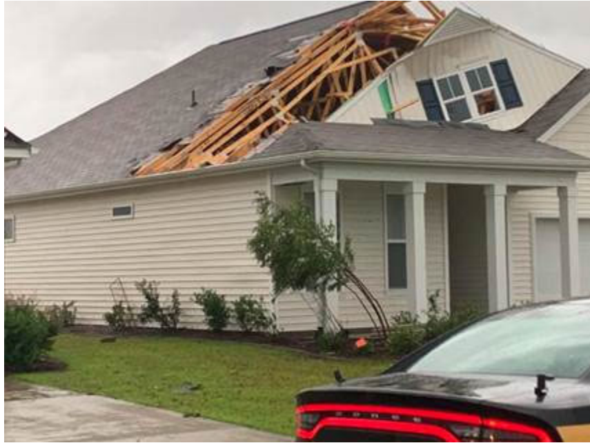
Figure 4.33. Failure of roof structure of single family home in Brunswick County, NC [Located approximately 33.921079, -78.576802] (Source: CNN )
