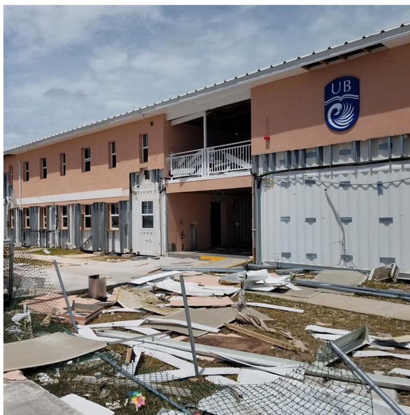
Figure 4.23. Wall cladding damage at the University of the Bahamas Northern Campus (Source: Dorothy Hall St. James ).
