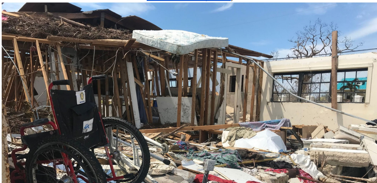
Figure 4.30. Wood-framed residential damage in High Rock, Bahamas. (Source: SkyNews )
