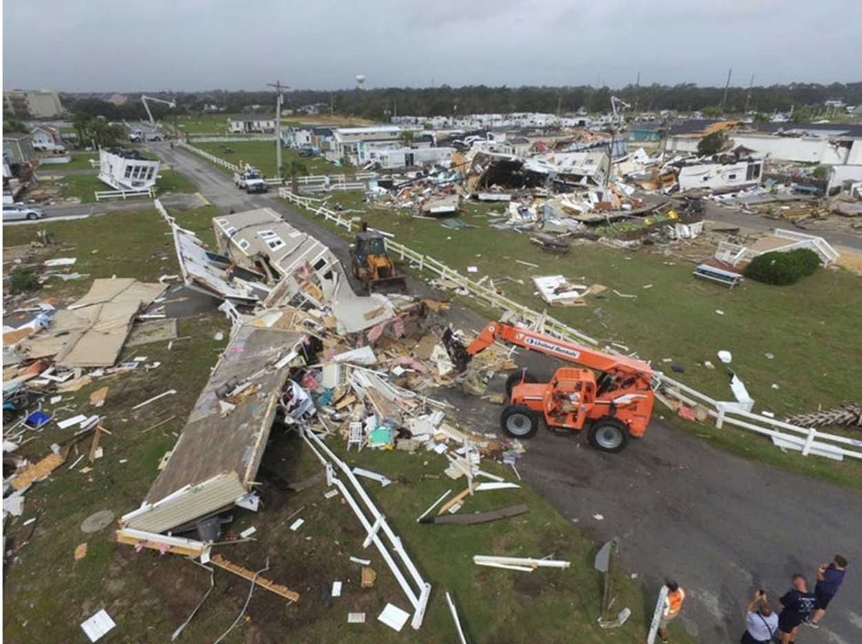
Figure 4.35. Boardwalk RV park in Emerald Isle, NC damaged by a tornado induced by Hurricane Dorian (Source: Patch.com ). From available photographs, the RVs had minimal anchorage to resist the tornado-induced winds.
