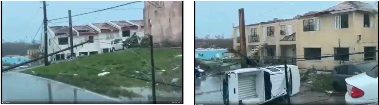
Figure 4.17. Damage to roofs of multi-family residential construction in Cooper's Town in North Abaco District of Abaco Island. (Source: https://twitter.com/i/status/1168701649847820289 , Footage by Amanda Degregory)
