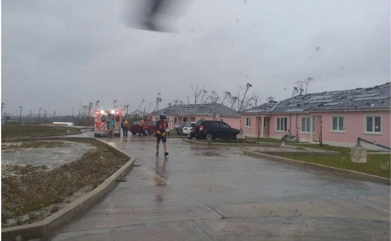
Figure 4.10. Roof cover loss at accessory buildings at Marsh Harbour Healthcare Center accessory structures [Located at 26.534, -77.070]. Note the snapped light pole in the foreground (Source: https://twitter.com/StevenCejas/status/1168910504183652353 )
