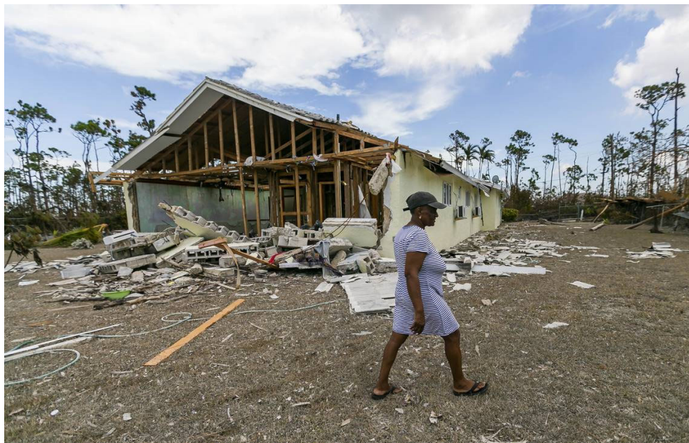
Figure 4.22. Unreinforced concrete block wall blowout in Freeport (Source: Matias J. Ochner/Miami Herald ).
