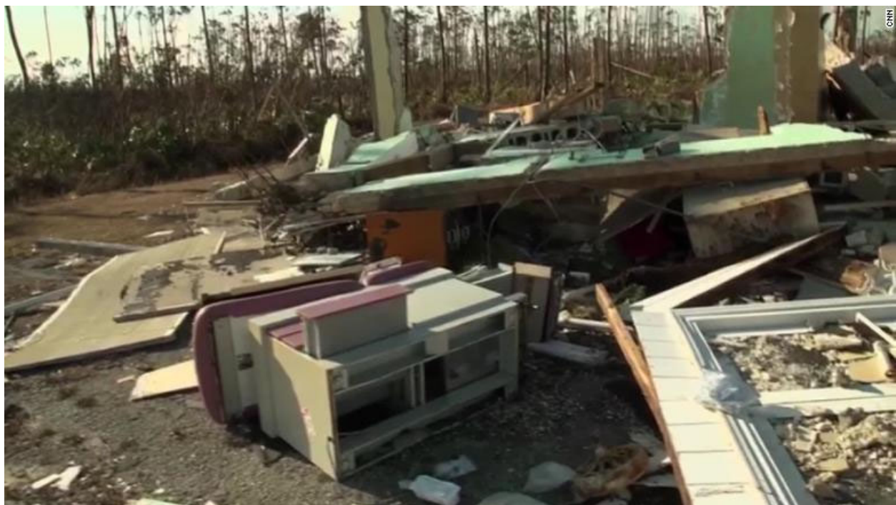
Fig. 4.28 Total building collapse of clinic in High Rock, Bahamas. Source: CNN
