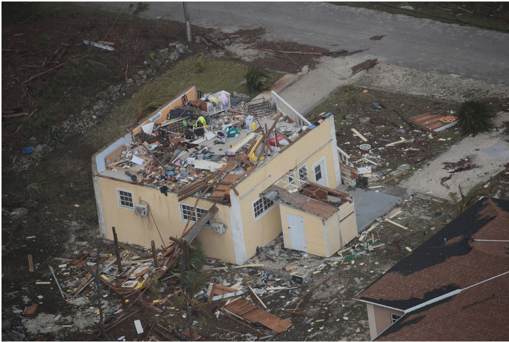
Figure 4.20. Failed roof and partial failure of upper story walls of residential structure in Freeport (Source: Scott Olson/Getty Images/Vox )
