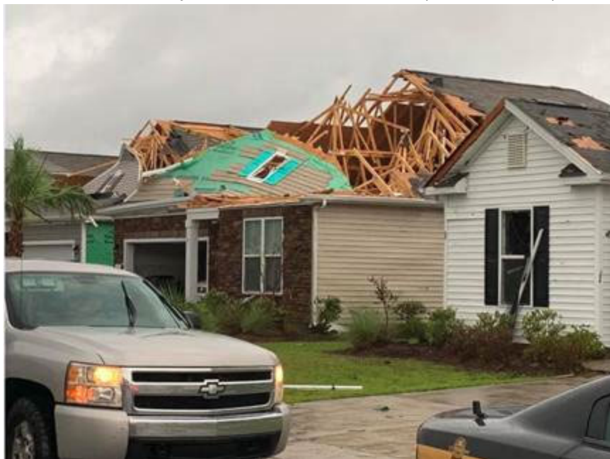
Figure 4.34. Envelope and structural damage to a row of single family homes in Brunswick, NC [Located approximately 33.921079, -78.576802] (Source: CNN )
