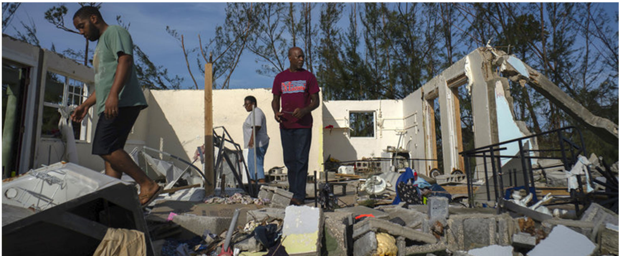
Figure 4.21. Remains of an unreinforced concrete block masonry single-family dwelling destroyed in the Pine Bay neighborhood of Freeport on Grand Bahama Island (Source: NPR )
