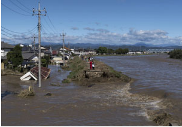
Figure 6: Floodwater flow through a break in the riverbank of the Akiyama River in Sano, Tochigi (left, The Atlantic, 2019), flood-damaged homes in Nagano (right, CNN, 2019a).
