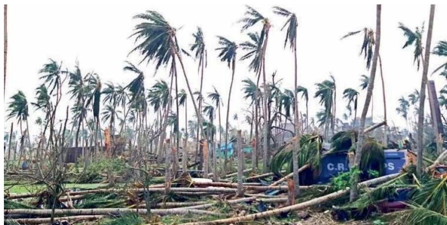
Ripped off coconut farms in Puri District.
