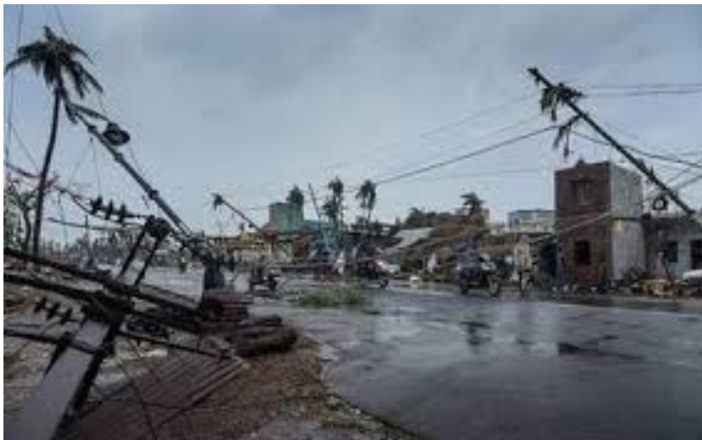
Aftermath of Cyclone, Devastation of electrical infrastructure
