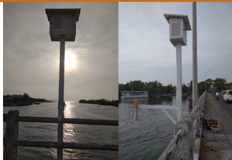
Figure 2. Water level gauge at Mattakkuliya
