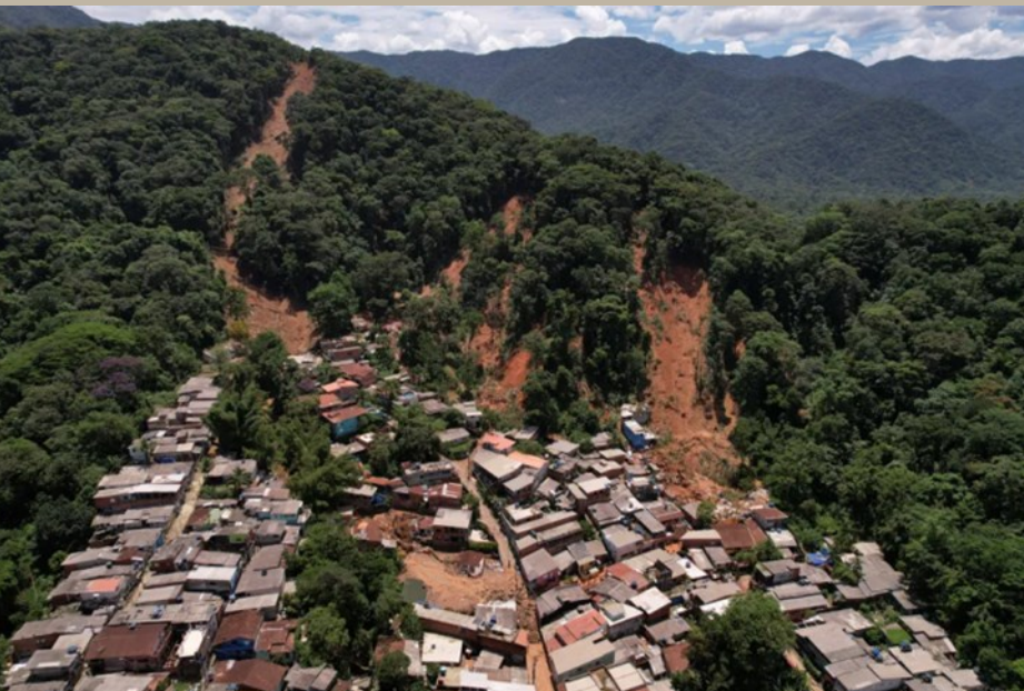
Figure 5 – Typical locality of simple houses just beside hillslopes in São Sebastião in February 2023 (Source: Amanda Perobelli/ Reuters)
