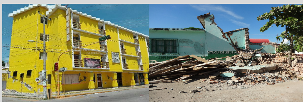
Structural damage in Juchitan, Oaxaca.
