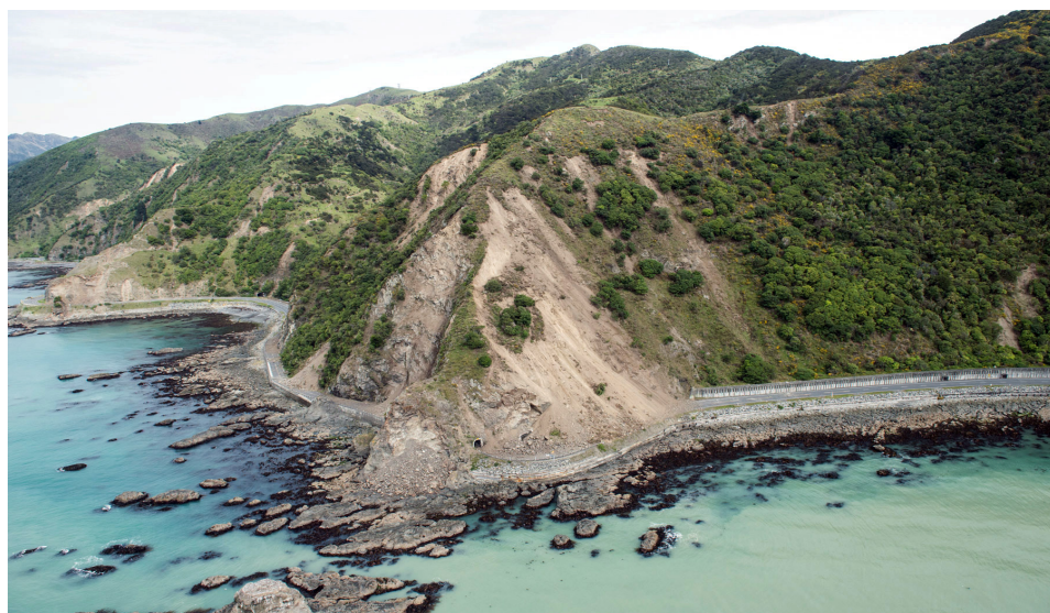
Fig. 1. Severed coastal highway system following Nov. 2016 Earthquake
