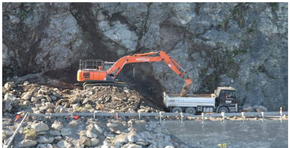
Fig. 3. Further damage to coastal highway following Cyclone Cook in April 2017
