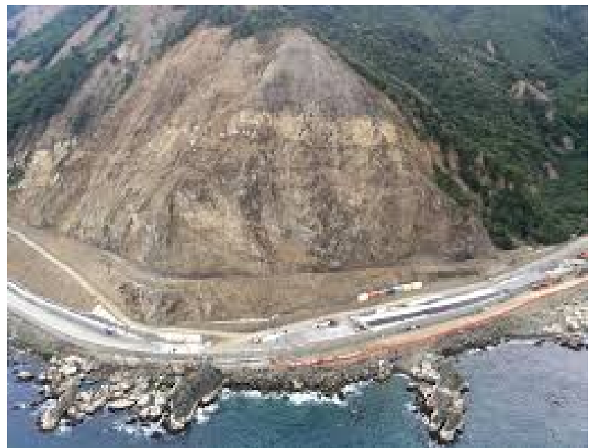
Fig. 2. Highway repairs late 2016
