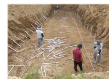
Photo 3. Installation of sensors into levee
