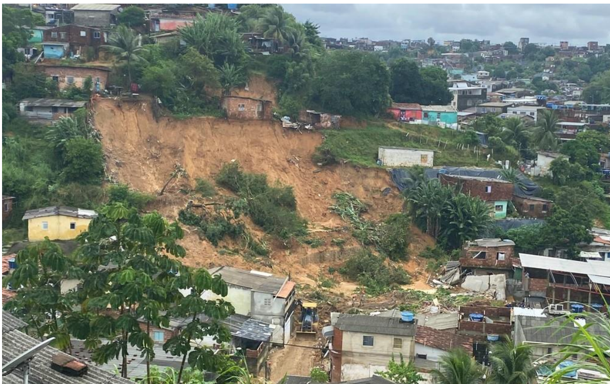
Figure 2 – Shallow landslide at the border between the municipalities of Recife and Jaboatão dos Guararape, Brazil, in May 2022 (Source: Alves, 2022)
