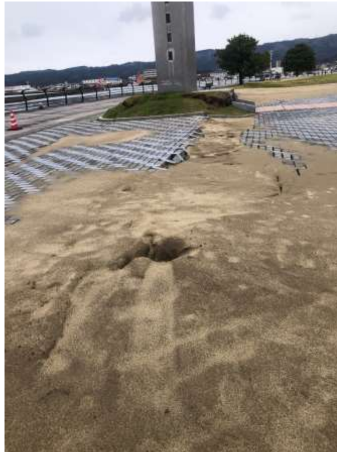
Sand ejecta and ground subsidence
