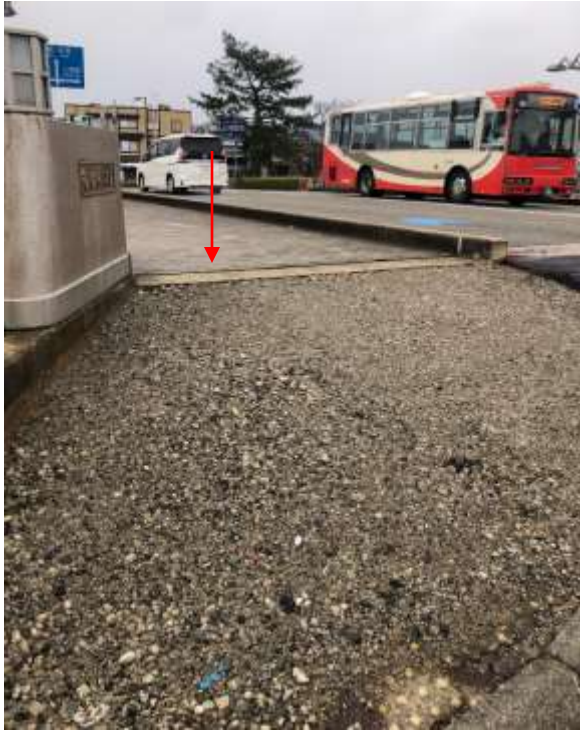
Ramp built to access bridge
