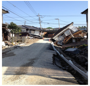
Photo 10: Collapsed houses in Mashiki Town, note ground failure, May 1, 2016
