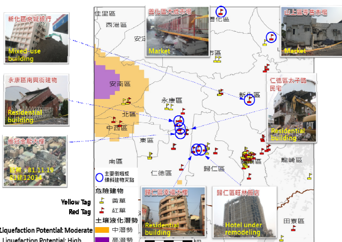
Locations of eight severely damaged buildings Source: NCDR
