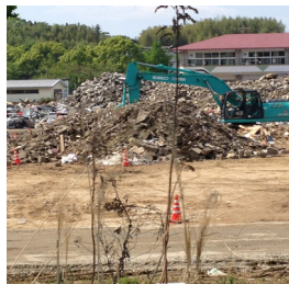
Photo 4: Separating debris at temporary dumpsite
