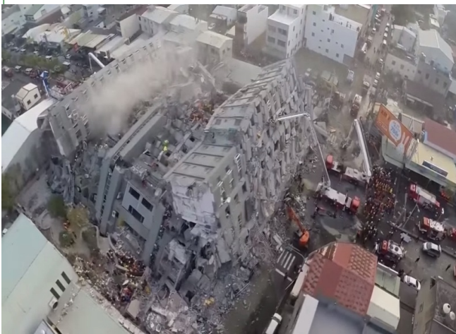
The collapsed Weiguan Jinlong Building
