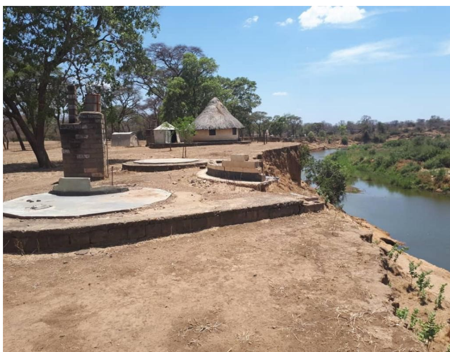
Figure 1: Tsetsefly research building structures that are threatened by gully erosion in Mbire Zimbabwe.
